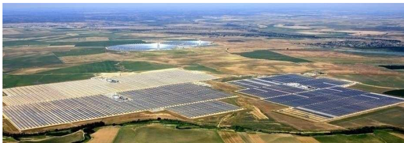
The first three units of Solnova in the foreground, with the two towers of the PS10 and PS20 solar power stations in the background.
